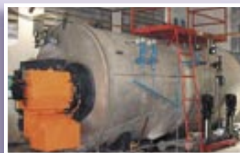
Trinuggal Garment Factory (Indonesia): 10 Tons Steam Boiler
